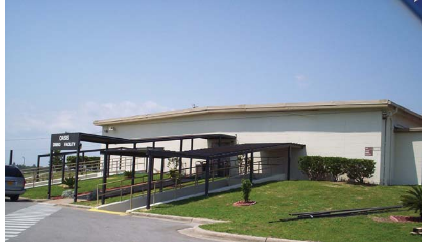
The Mole Hole, in its Current use as a Dining Facility. Source: Eglin Air Force Base, Cultural Resources Division.
