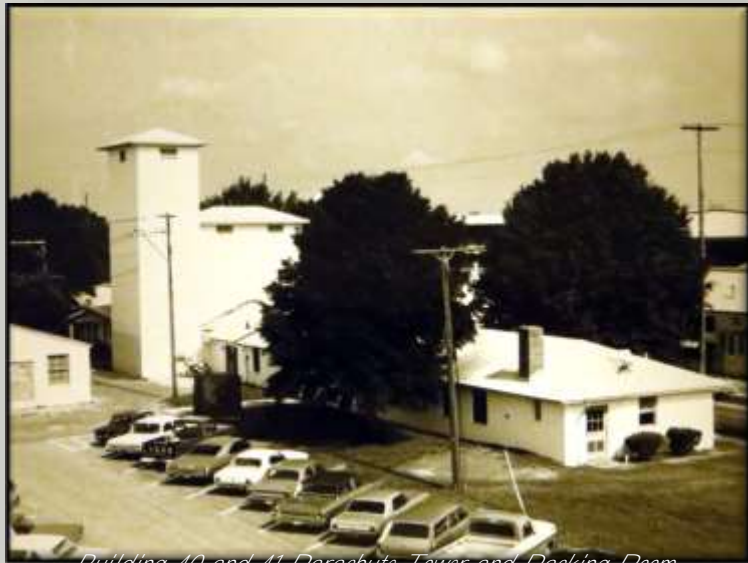
Building 40 and 41 Parachute Tower and Packing Room
