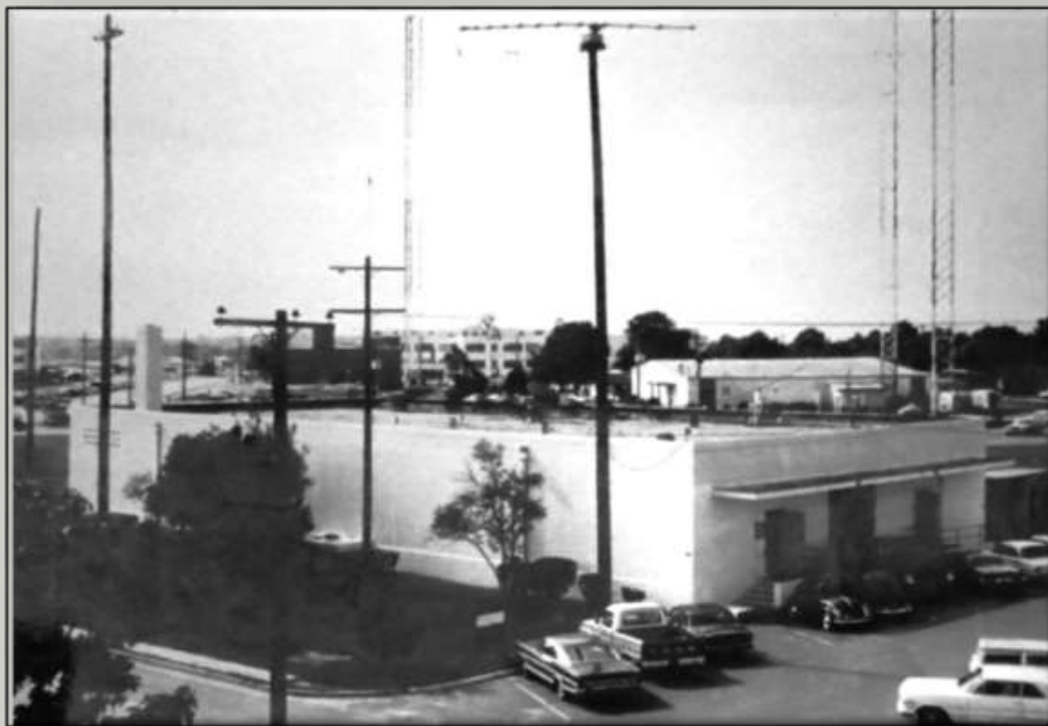
Building 44 Armament Instrument and Inspection Building
