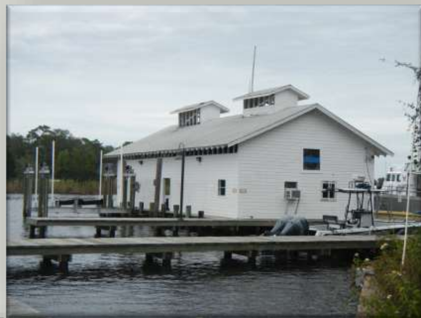
Marine Operations Building on Weekly Bayou
