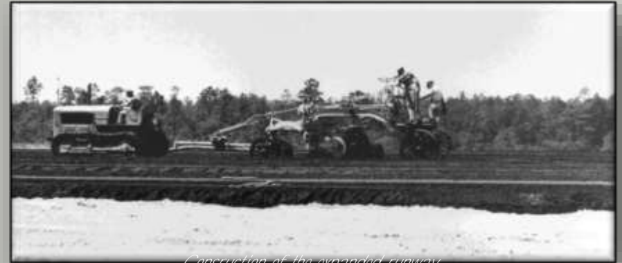
Construction of the expanded runway
