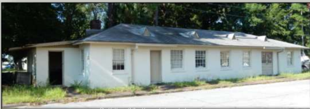
Building 30 oil, paint and dope storage
