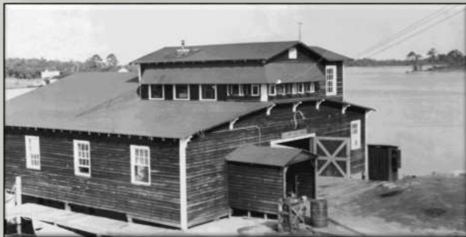
Marine Operations Building on Weekly Bayou
