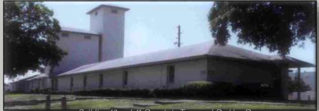
Building 40 and 41 Parachute Tower and Packing Room
